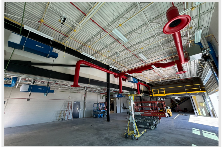
Photo of the various colors being painted on to identify the different MEPF systems being installed at the Skills Lab Addition.
